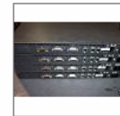
Cisco 2503 Router Lot of 4 Units Powered Up, Good Fans.
